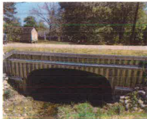
Figure 6-Mill Creek Drive Replacement Culvert
